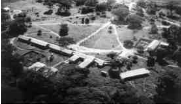
Das Wasso Hospital 1976
